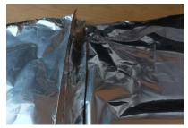
Lift the overlap and crease for the full 65 cm length of the seam
