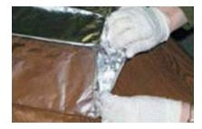
Roll the ends twice and press flat against the foam block
