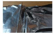
Lift the overlap and crease for the full 65 cm length of the seam
